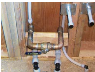
House water shut off under cabinet..
