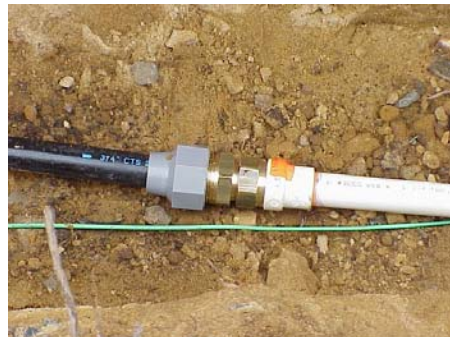
Connection of CPVC to Polybutylene. Polybutylene is to be used outside only. The black pipe.
