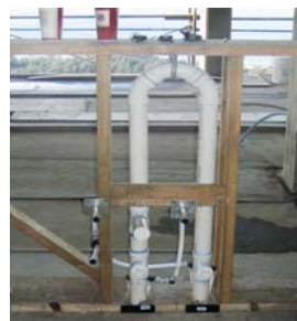
Loop vent to top of cabinet
