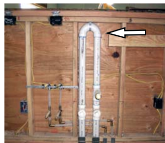
Rough in of loop vent and water
