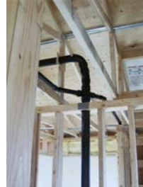
Vents connecting together in attic.
