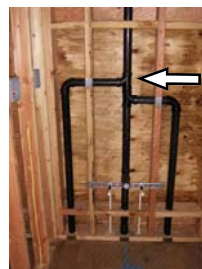
Vent connection of downstairs fixtures must be 6" above the overflow rims of fixtures on this floor.
