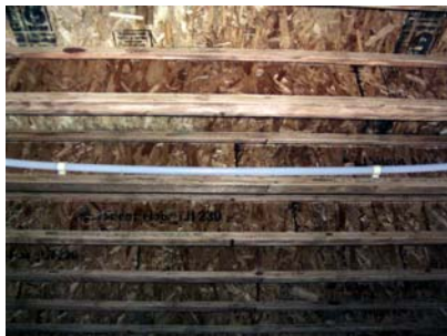
Strap water pipe using chart above.
