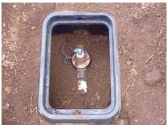
With water pressure over 80 psi a pressure regulator is required.
