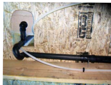
Bath tub drain with flat vent. Looking up at second floor, floor joist.
