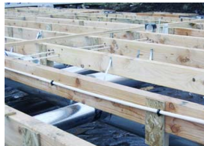
Under floor pipe up in joist space where it will be insulated
