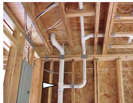
Waste connection downstream of toilet
