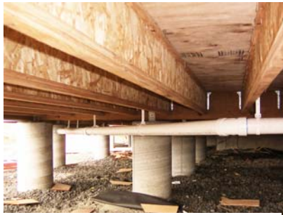
Hang ABS or PVC waste pipe at 4 foot on center.
