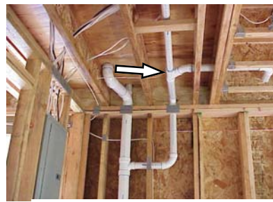
Combination y-1/8 bend in horizontal position.
