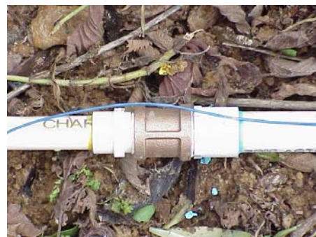
Connection of PVC to CPVC outside of house. PVC is not allowed to be inside of house.
