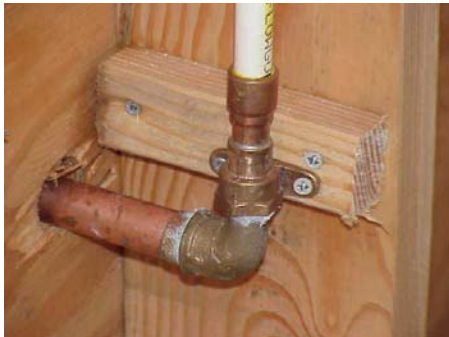
Flow Guard gold CPVC water pipe fastened to structure for hose bib outside.
