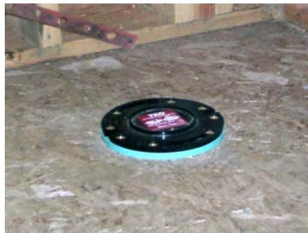
Toilet flange with brass screws holding it to floor. Cap for test. Blue spacer ring for sub sheeting.
