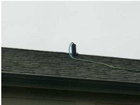
Hose in roof vent filling waste with water for test. Ten foot head of water.
