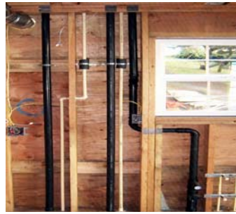
Mid-story strap waste, vents and water lines.
