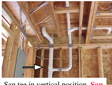
San tee in vertical position. San tee in horizontal position not permitted as drainage fitting.
