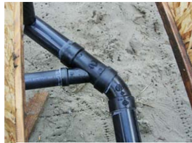
Y-fitting receiving waste from sink.
