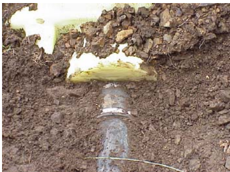
Connection of ABS waste pipe to septic tank using a Fernco rubber coupling.
