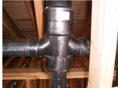
Double san tee. Used to connect two horizontal vents to a vertical stack. Fitting upside down.
