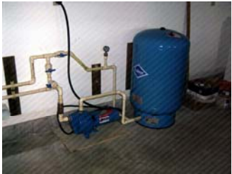
.Water pressure can be increased with a well pump and bellows tank.
