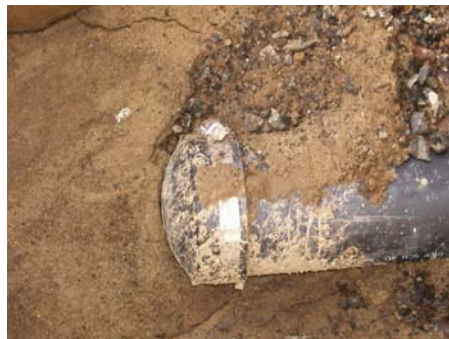
Test cap on sewer line.
