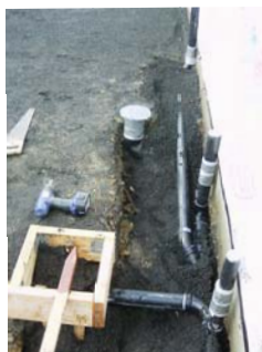
Shower access box in concrete floor.
