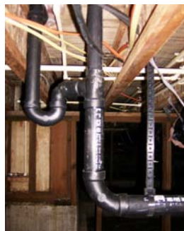
Bath tub drain with vertical vent.
